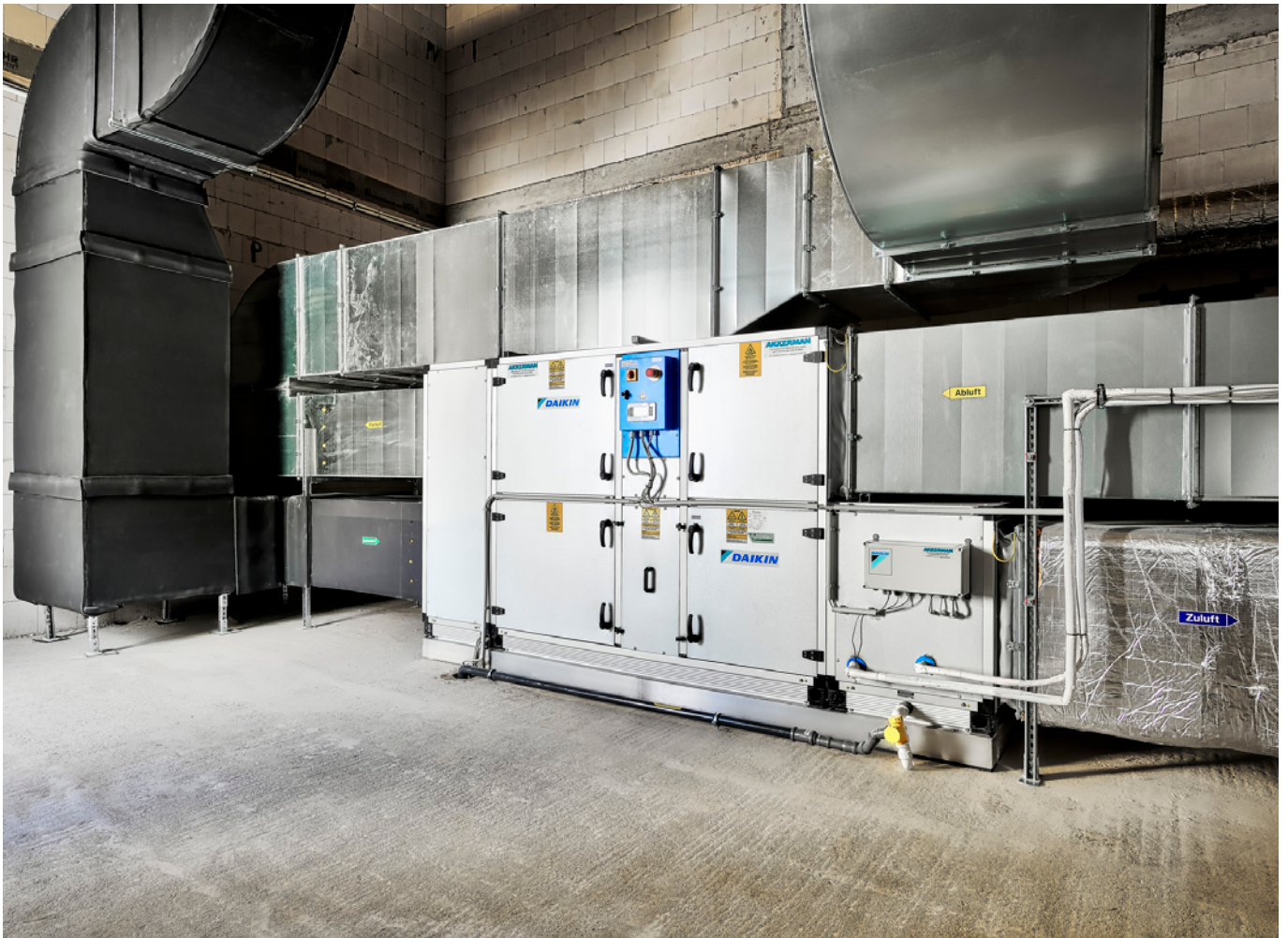
D-AHU Modular R installation
