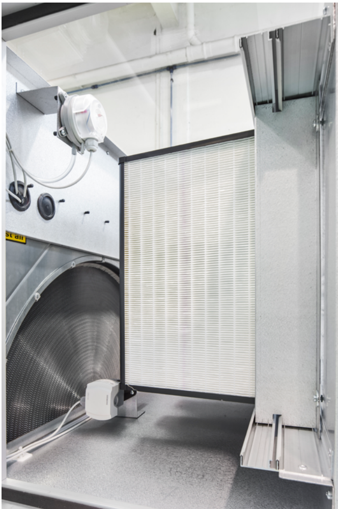
Heat recovery wheel and filter
