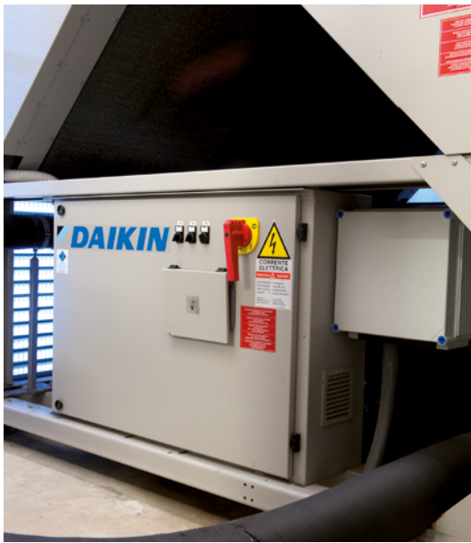
Air cooled chiller installation
