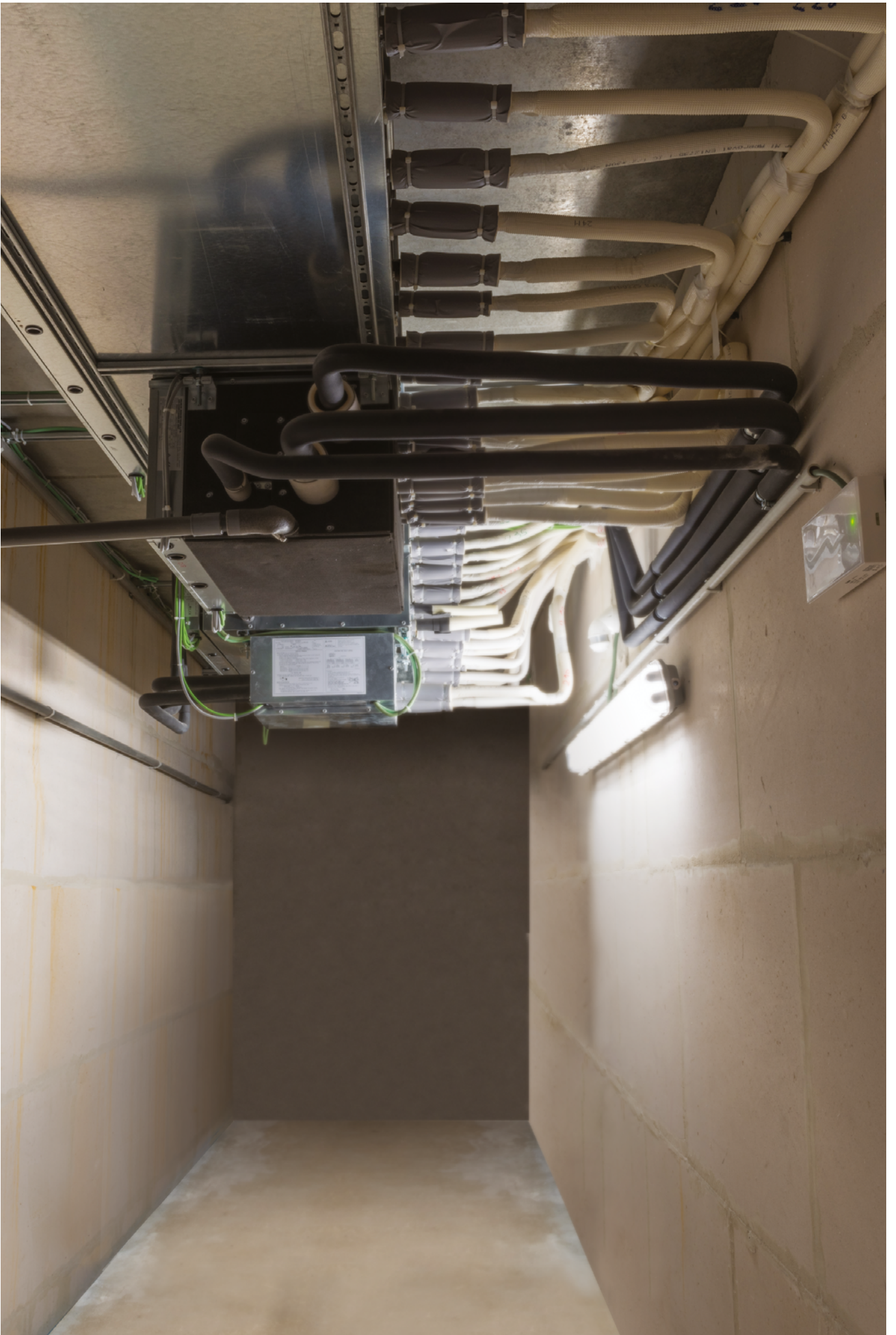
Individual and multi branch selector box installation
