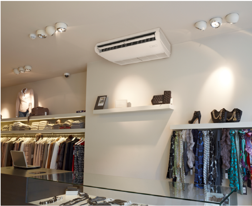
Ceiling suspended unit
